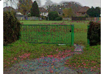
Existing gate and fence to be switched around so gate is located at the end of the new footpath. This to be organised by Water Orton Parish Council.
